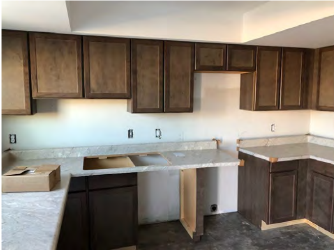
Preservation Square, Phase I
