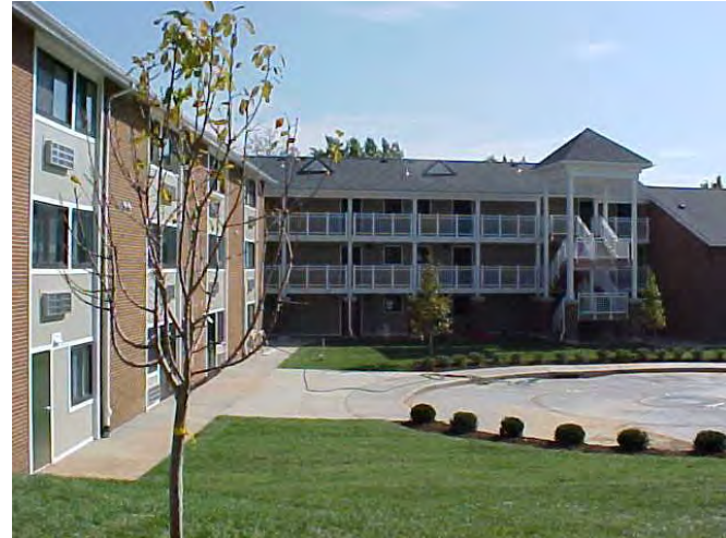
Badenhaus Sewer Improvements
