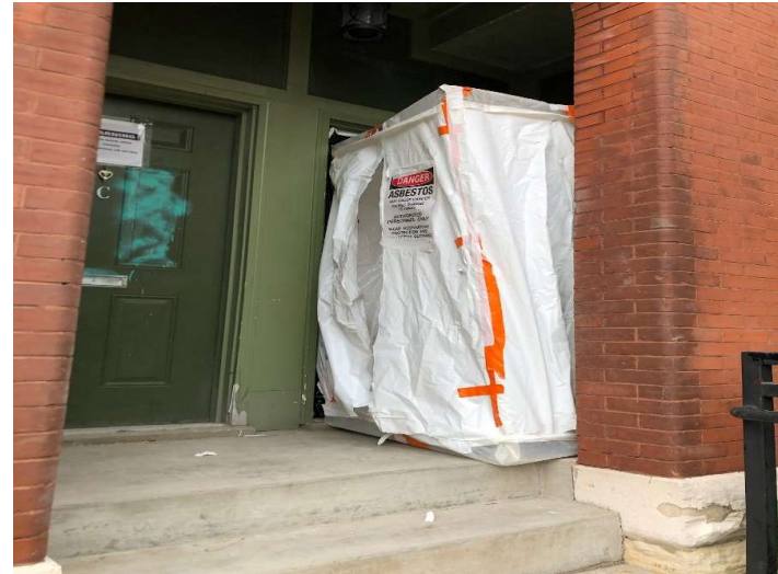
2900 Park Structural Repairs & Unit Upgrades
