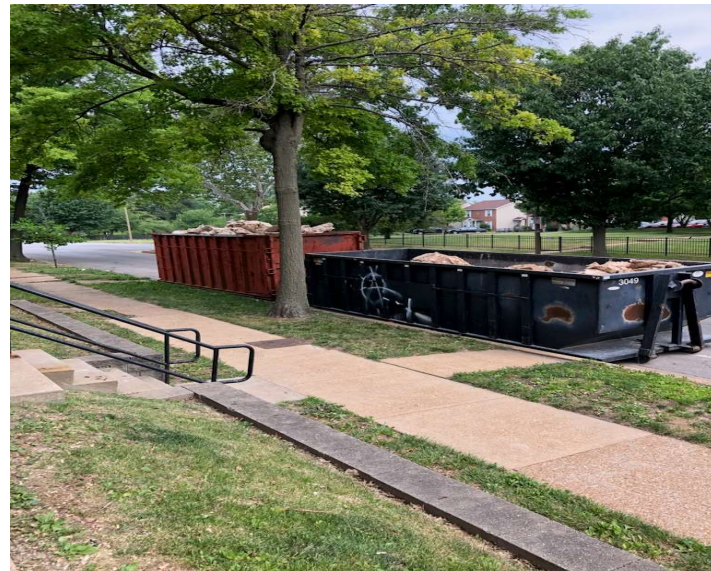
2900 Park Structural Repairs & Unit Upgrades
