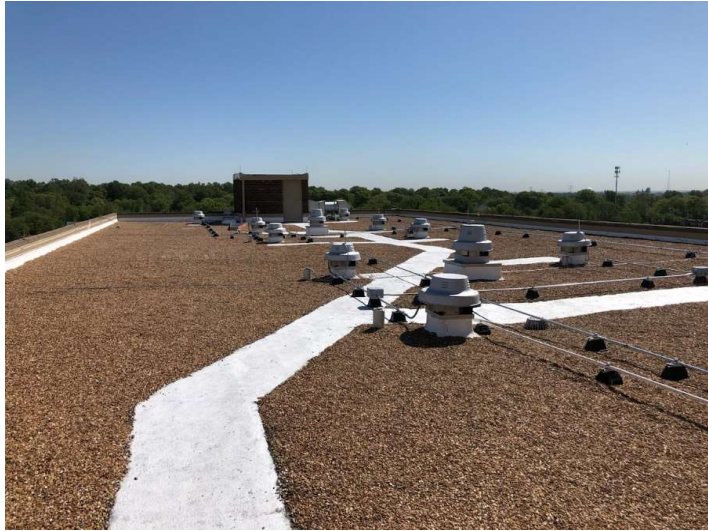
Euclid Roof Replacement & Exterior Building Repairs
