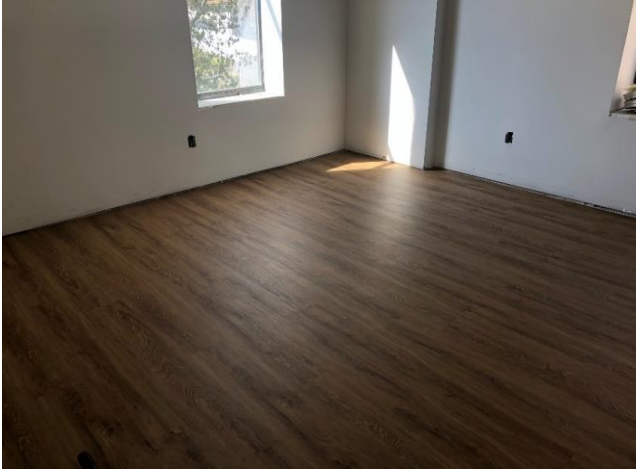
2900 Park Structural Repairs & Unit Upgrades
