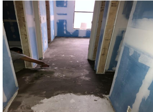
2900 Park Structural Repairs & Unit Upgrades
