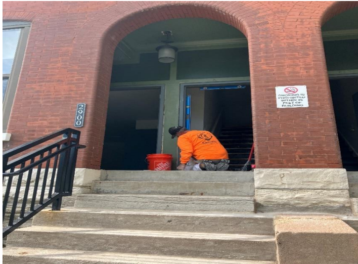
2900 Park Structural Repairs & Unit Upgrades
