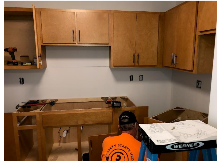
2900 Park Structural Repairs & Unit Upgrades
