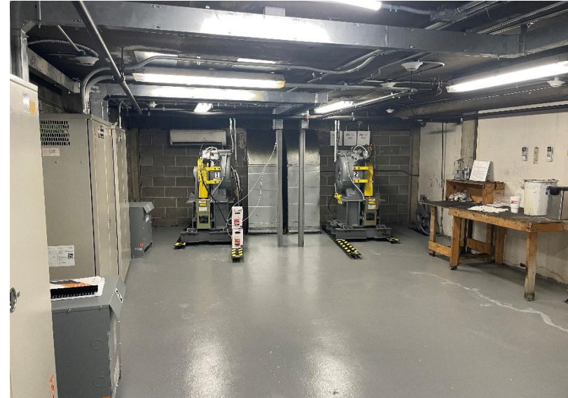
Parkview Elevator Replacment
