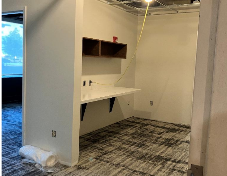
Parkview First Floor Renovations
