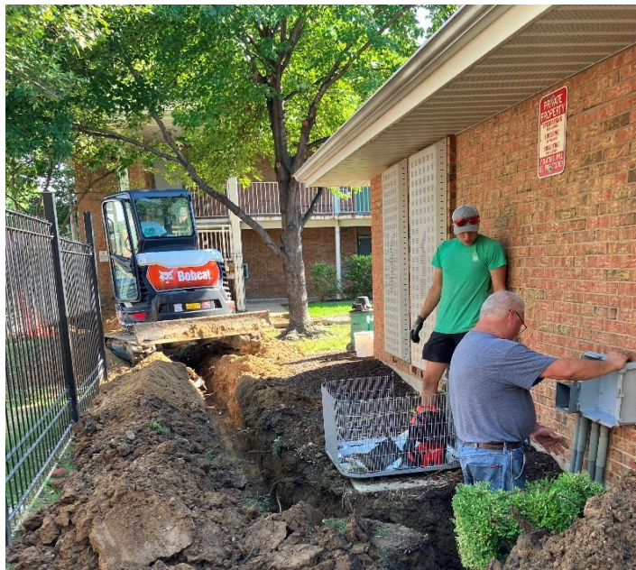
California Gardens Security Fence & Stair Repairs
