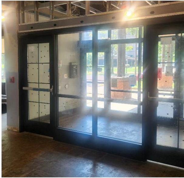
Parkview First Floor Renovations
