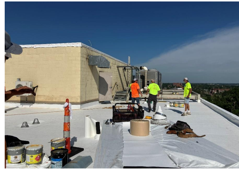
James House Emergency Roof Replacement
