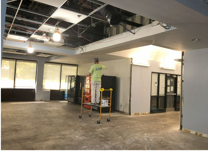
Parkview First Floor Renovations
