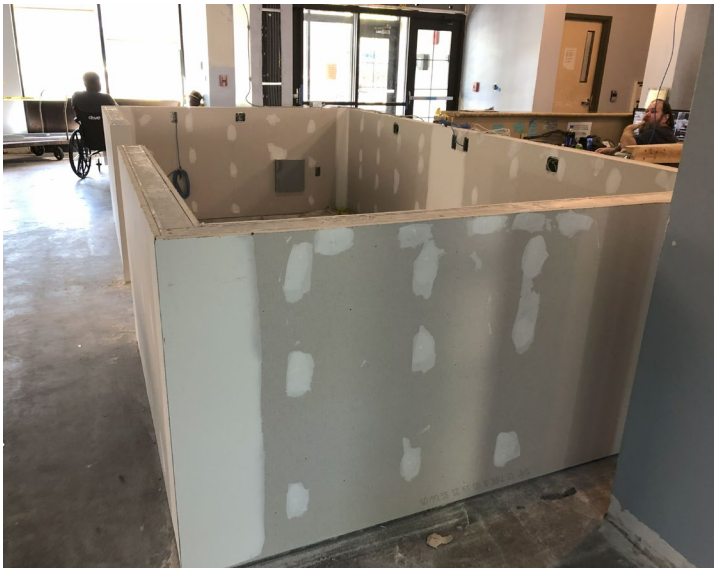
Parkview First Floor Renovations
