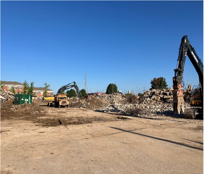
Clinton-Peabody Redevelopment - Phase 1 Demo
