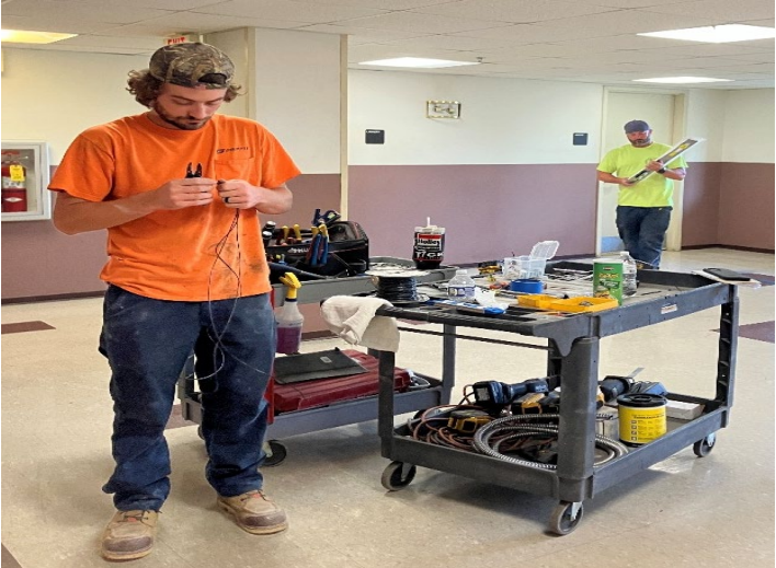
West Pine Elevator Replacement
