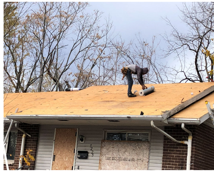
Asphalt Roof Replacement
