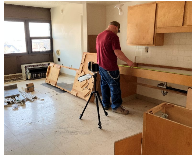
Parkview Unit Repairs
