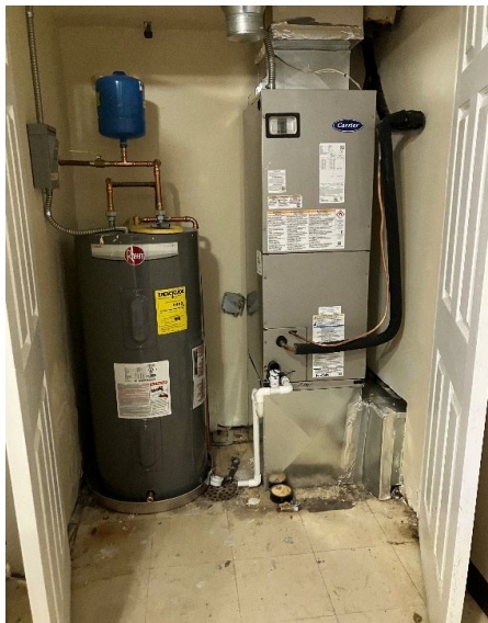
NSSS Electrification & Unit Repairs (Towne XV)
