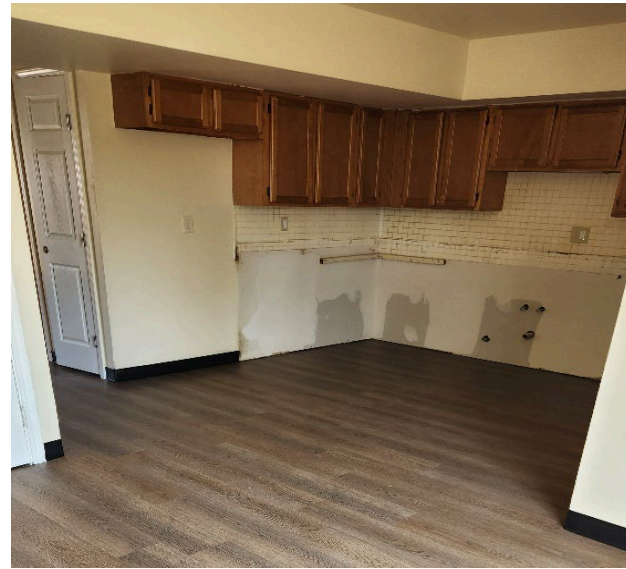
Lookaway Unit Repairs
