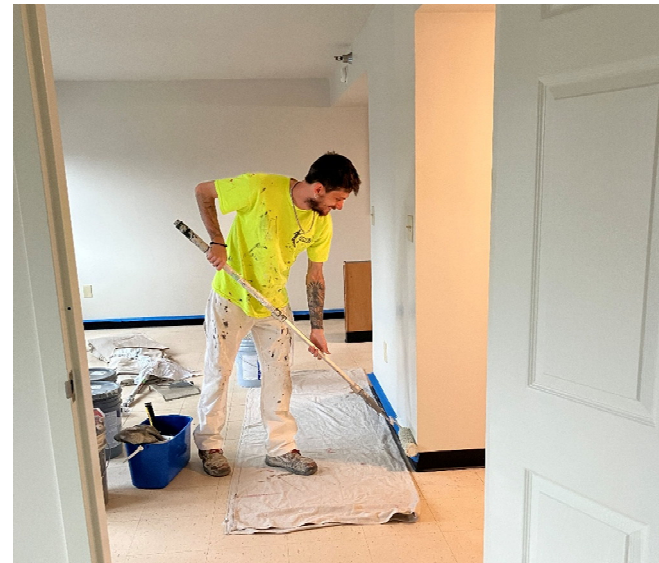
Parkview Unit Repairs
