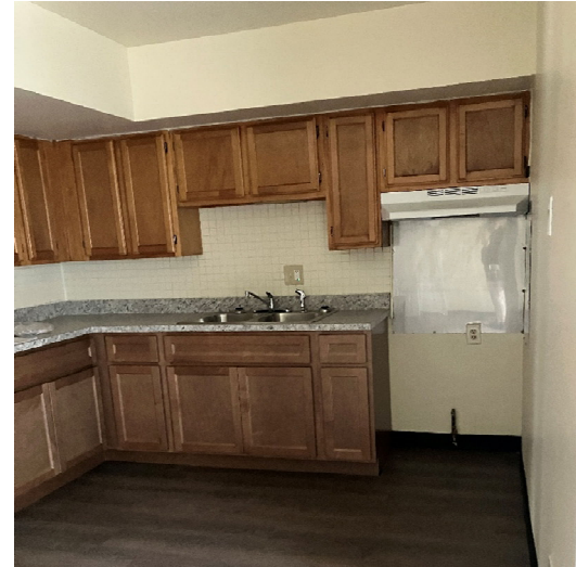
Lookaway Unit Repairs
