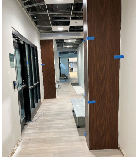
Parkview First Floor Renovations
