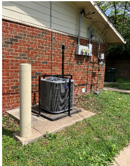
NSSS Electrification & Unit Repairs (Towne XV)
