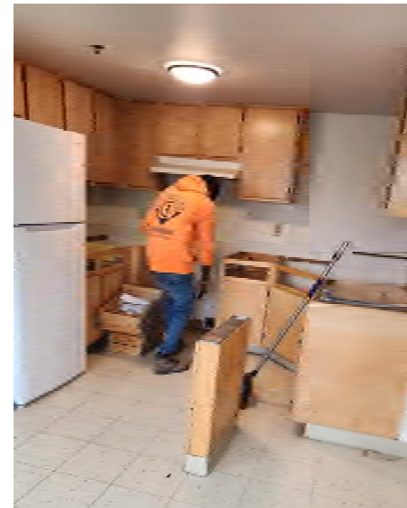
Parkview Unit Repairs
