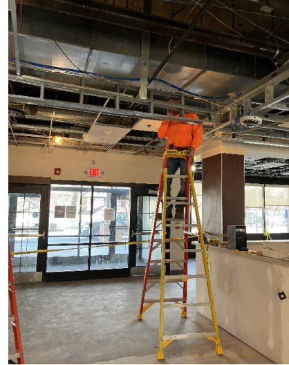
Parkview First Floor Renovations
