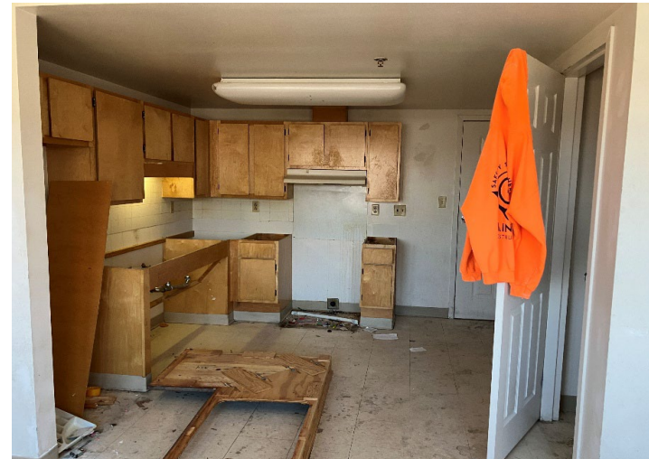
Parkview Unit Repairs
