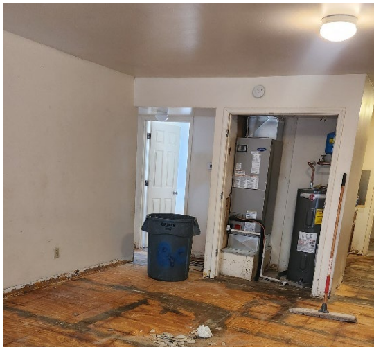
NSSS Electricification & Unit Repairs (Samuel Shepard)
