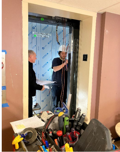
West Pine Elevator Replacement
