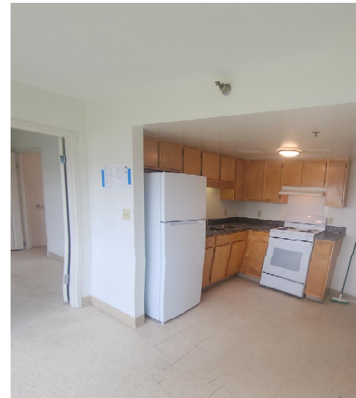
Parkview Unit Repairs
