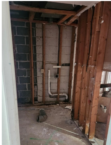
NSSS Electrification & Unit Repairs (Page Manor)
