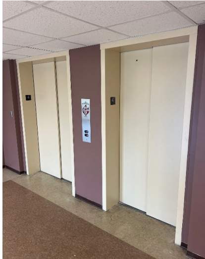
West Pine Elevator Replacement
