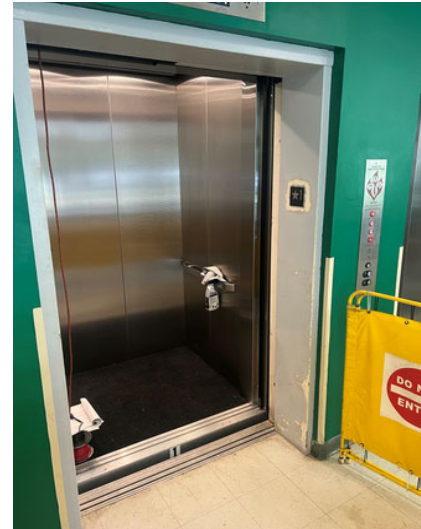
West Pine Elevator Replacement
