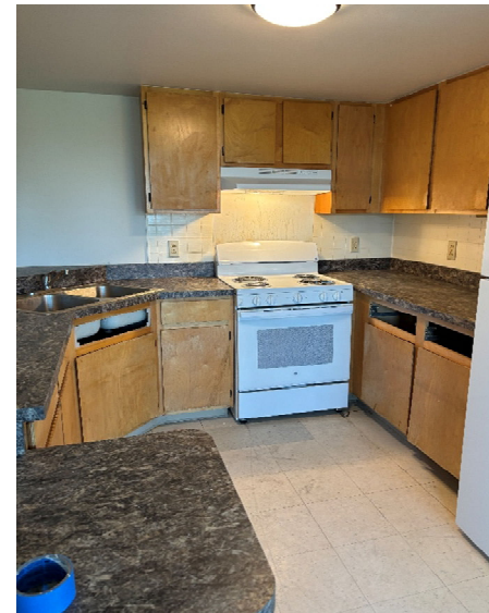
Parkview Unit Repairs
