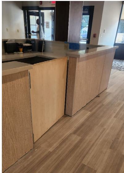
Parkview First Floor Renovation
