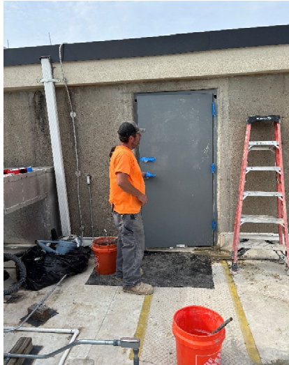
West Pine Elevator Replacement
