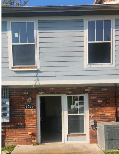
McMillan Manor I Unit Repairs
