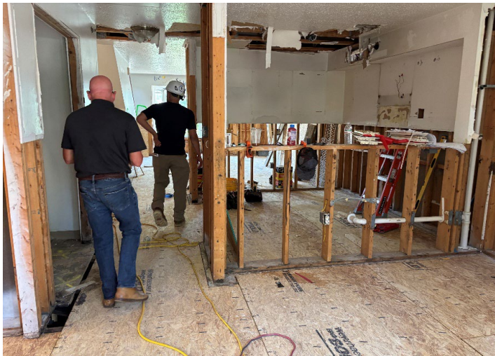
McMillan Manor II Unit Repairs
