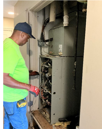
McMillan Manor I Unit Repairs
