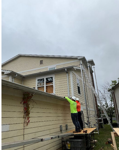
McMillan Manor II Unit Repairs
